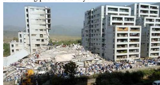
b) Failure of irregular building in Islamabad [8]
